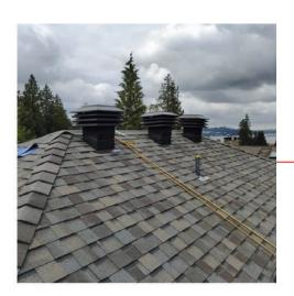
The Roofing Contractors Association of BC (RCABC) says, "Attic ventilation is not the responsibility of the roofing contractor as it is a design and building code requirement." Shingle manufacturers also say that without proper ventilation, their warranties become void.
