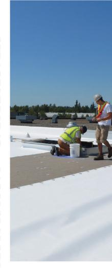
Your flat roof should never be perfectly flat. A perfectly flat roof has a risk of standing water, making drains ineffective. Standing water can shorten the lifespan of the membrane and add excessive weight to the roof which creates sagging, creating more standing water. To prevent this issue, a Slope Package can be installed on the roof to create a more efficient way for water to be directed towards the drains. This will effectively mitigate standing water problems.
